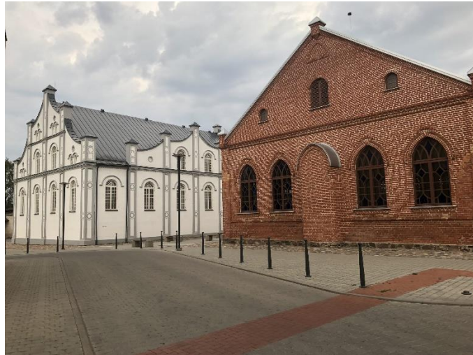
Picture 3. Joniškis Synagogue Complex, Lithuania. The White and Red Synagogues form a rare ensemble of two 19th-century brick synagogues, restored and adaptively reused for cultural and educational purposes while preserving the architectural and historical legacy of the town's Jewish community.
