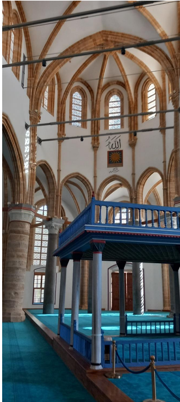
Picture 4. Interior of the Selimiye Mosque (former Cathedral of Saint Sophia), Nicosia, Cyprus. Built as a Latin Catholic cathedral in the 13th–14th centuries (ca. 1209–1326) in the French High Gothic style, it was converted into a mosque after the Ottoman conquest in 1571, while retaining much of its Gothic architectural fabric. The ribbed vaults and pointed arches remain largely intact, complemented by later Islamic elements such as the mihrab and mahfil. Conservation and restoration works in the Selimiye quarter, including the monument, have been supported by the European Union as part of broader cultural heritage preservation programmes in Nicosia.
